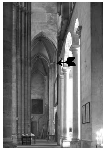
Lagny west wall of choir
