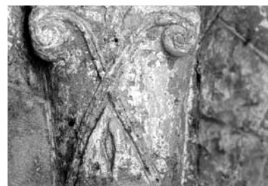
Bury nave aisle Ws4
